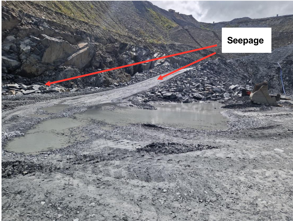
Figure 6-4 - Southern Wall and Ramp Seepages
