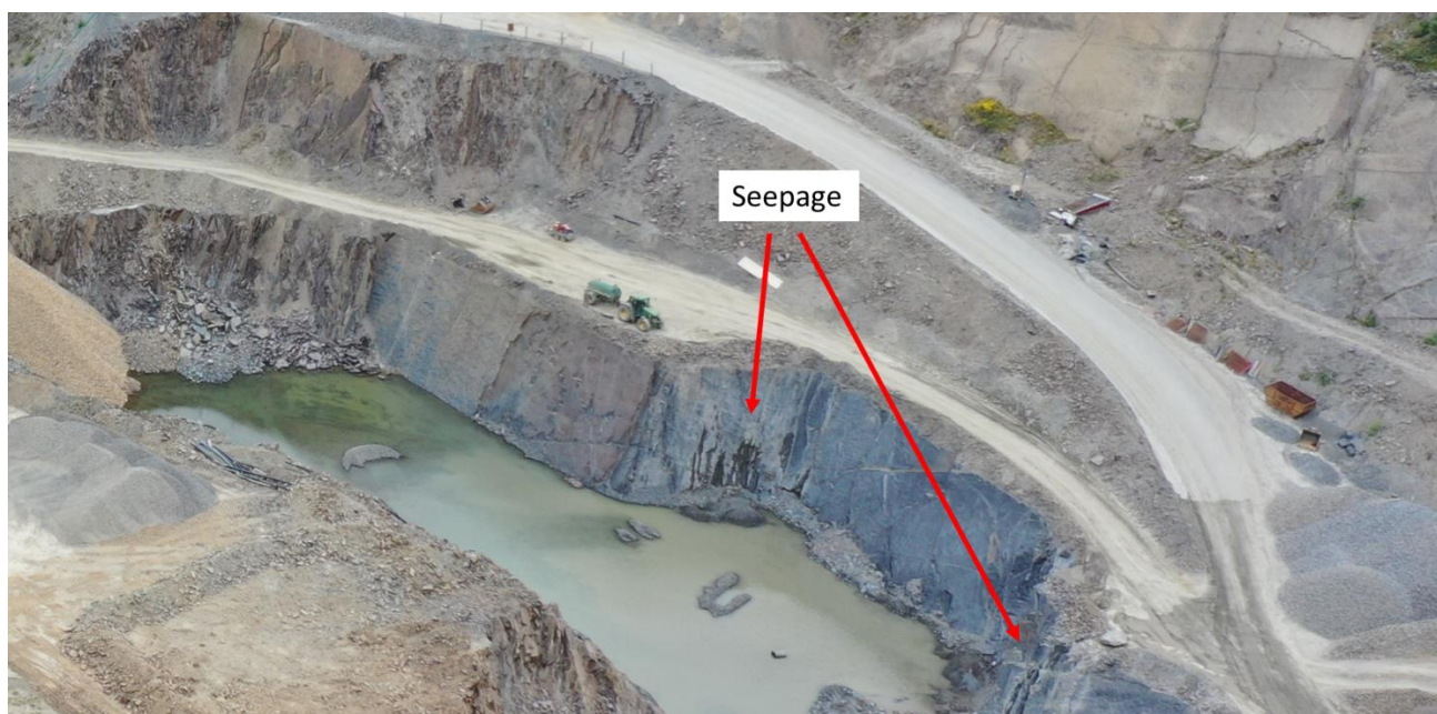
Figure 6-7: Seepage observed on western quarry wall ~240 mAOD (July 2019).
